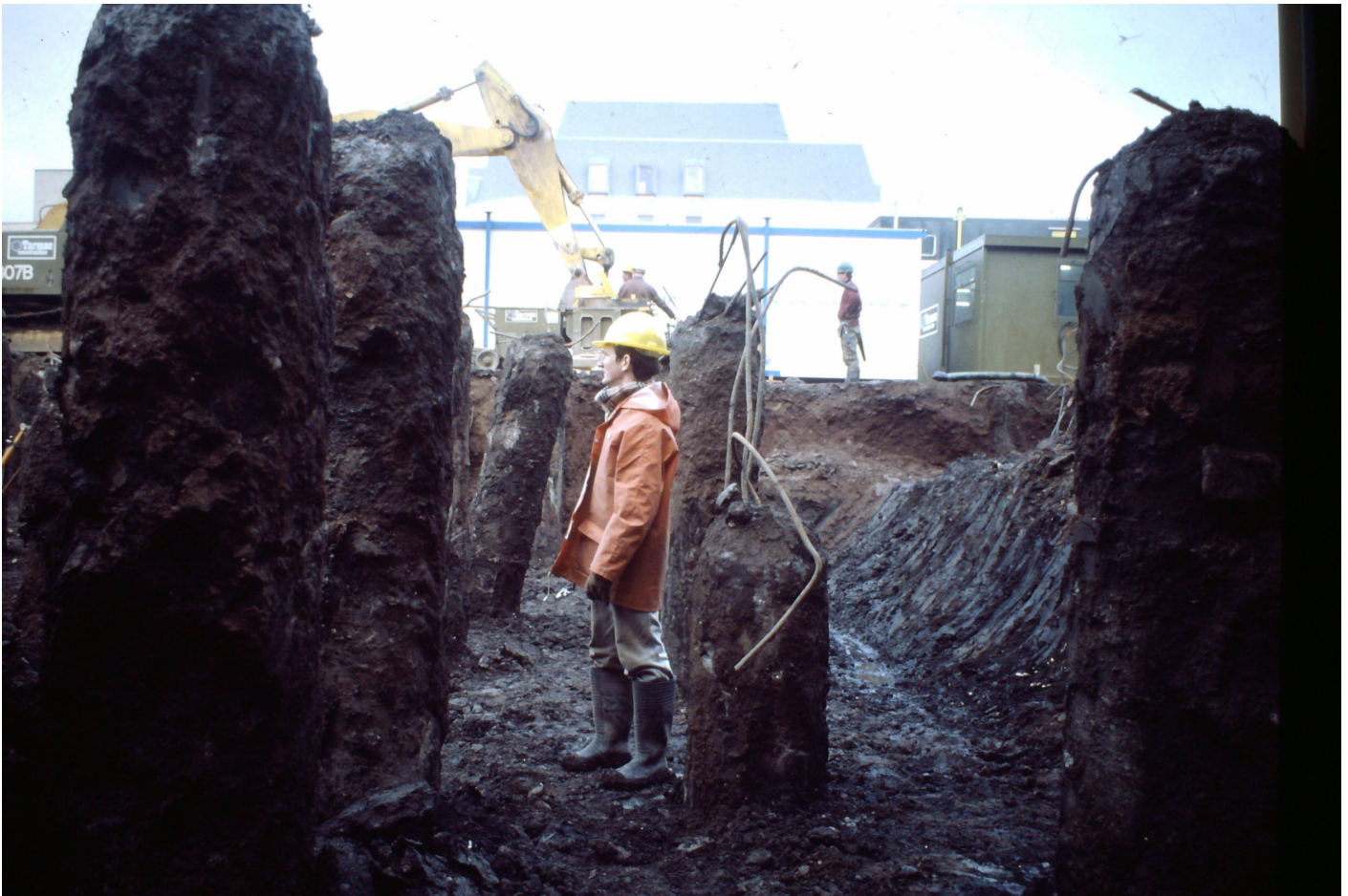
Undertaking a watching brief at St John's Square - Photo © ARO.
